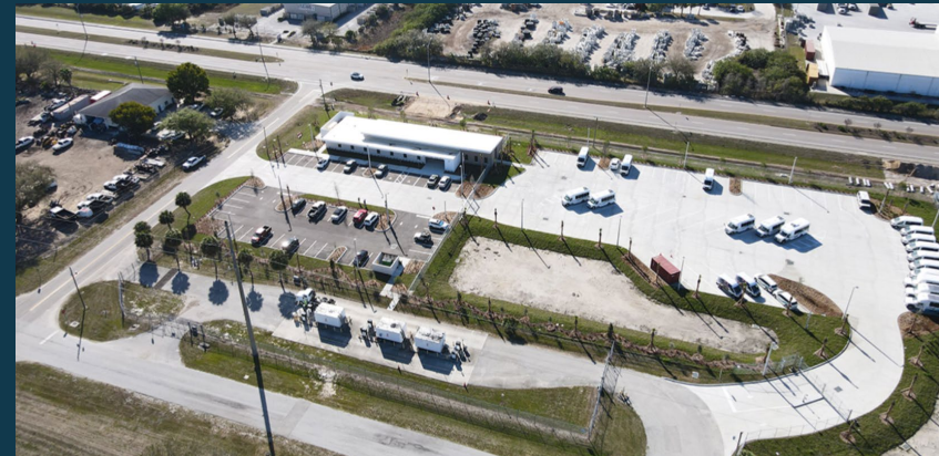
Charlotte County Transit Facility Charlotte, FL.
